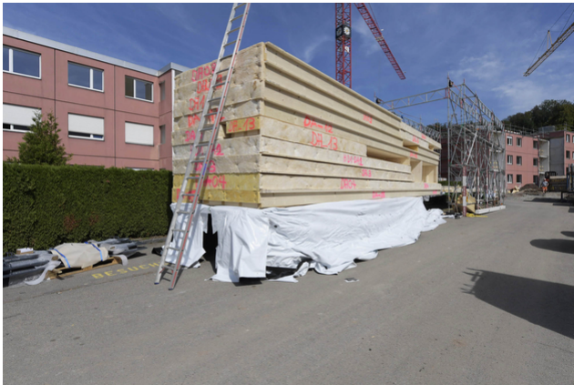
Delivery of the prefabricated wooden elements
