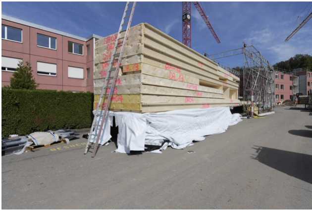
Delivery of the prefabricated wooden elements
