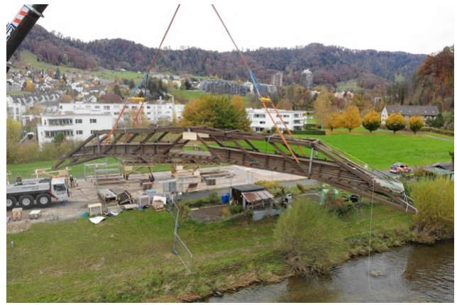
Assembly work on the bridge
