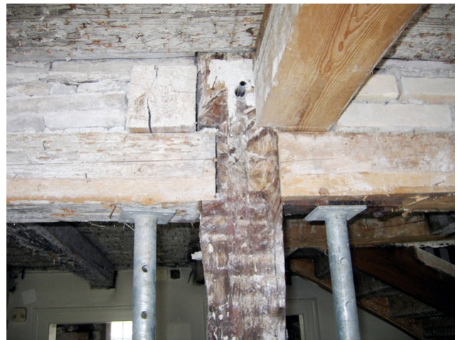
Support for beams on the first floor before renovation
