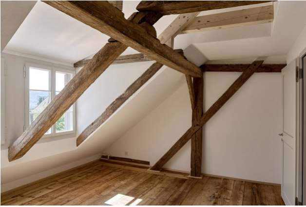
Existing roof truss
