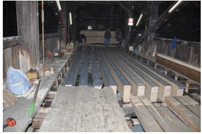
Assembly new side member at night
