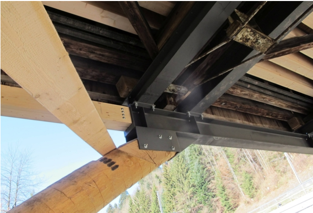
Connection of the oak logs and compression bars
