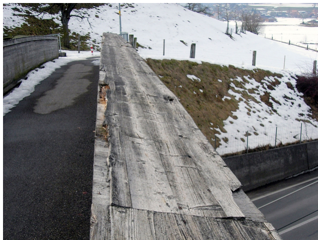
Pedestrian bridge before renovation 1
