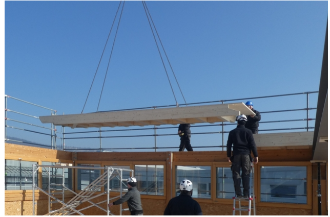
Installation of a roofing element
