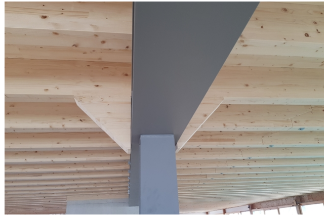
Combination of steel structure and wood construction
