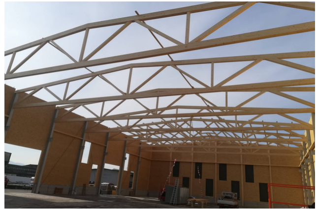
Assembly production hall
