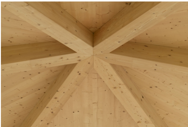
Roof soffit on cross-laminated timber with purlins converging in the center
