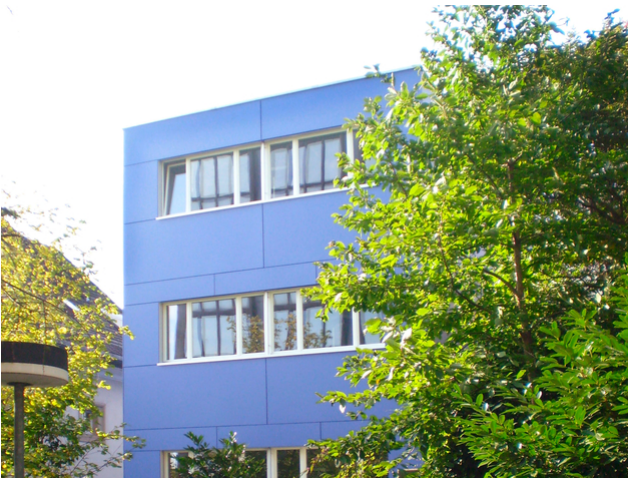
Facade narrow side
