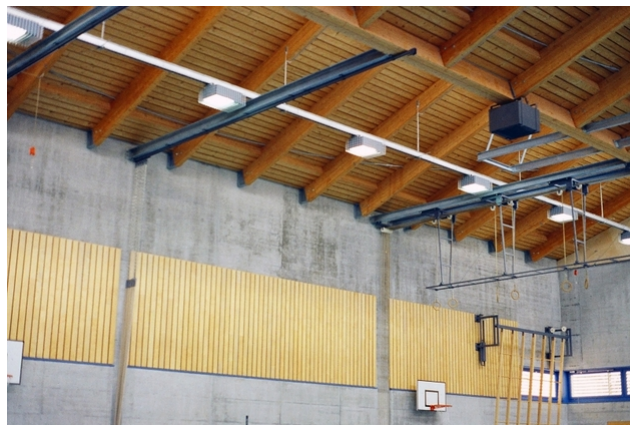
View of exposed rafter position
