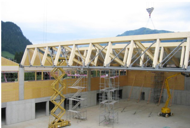
Assembly of lattice girders
