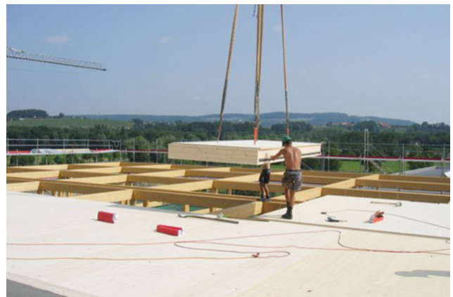
Assembly of roof elements
