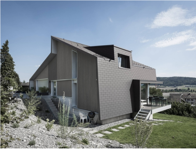
Special shape: The roof extends to the ground on one side
