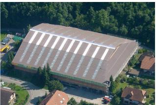
A roof for the previously open ice rink was to be built over the existing civil defense facility. The building lines allowed hardly any leeway in the design of the roof shape. Limitations had to be observed not only in the ground plan, but also in the section.
