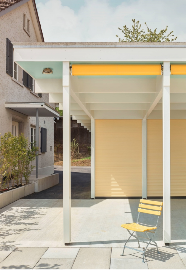
The supporting structure remains visible
