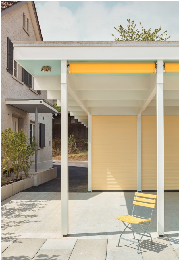
The supporting structure remains visible
