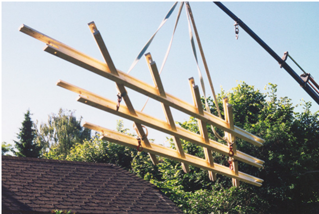
Unloading the beam grate
