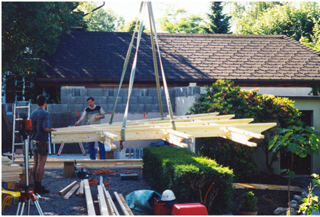
Lifting girder grid
