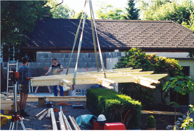
Lifting girder grid
