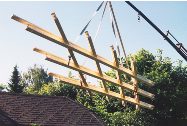
Unloading the beam grate
