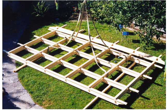
Fold out girder grid on flat surface and install edge and reinforcement girders
