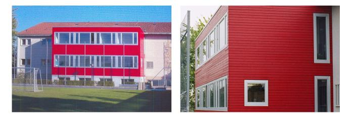
Here, a two-story rucksack addition to the existing building was to be realized, with adaptation of the existing eaves and transitions to the first building. The facade was to be created with a painted wooden formwork.
