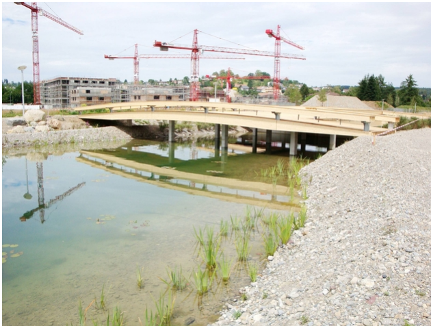
Bridge park access
