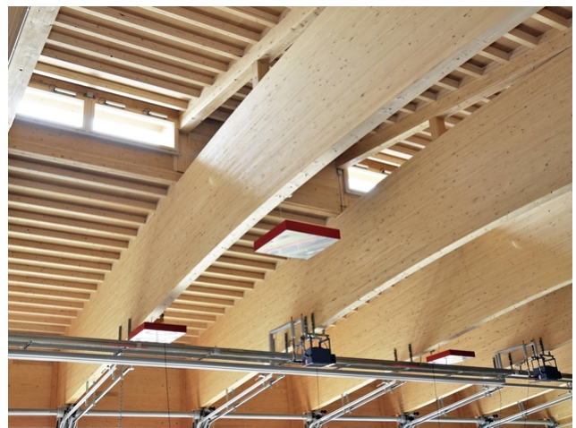
Detail of the large and heavy wooden arch trusses
