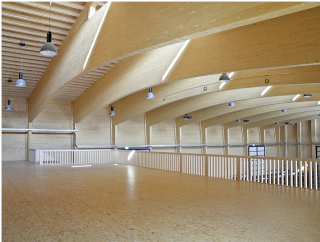
The Simmental Arena gallery: view of the arch trusses
