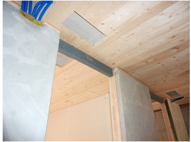
Wall coating as a heat accumulator
