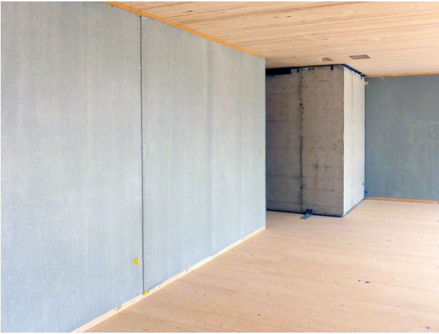
View wood concrete wall
