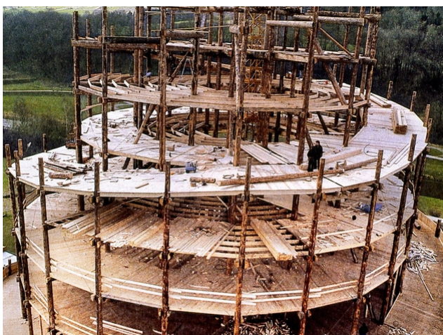
Tower in shell
