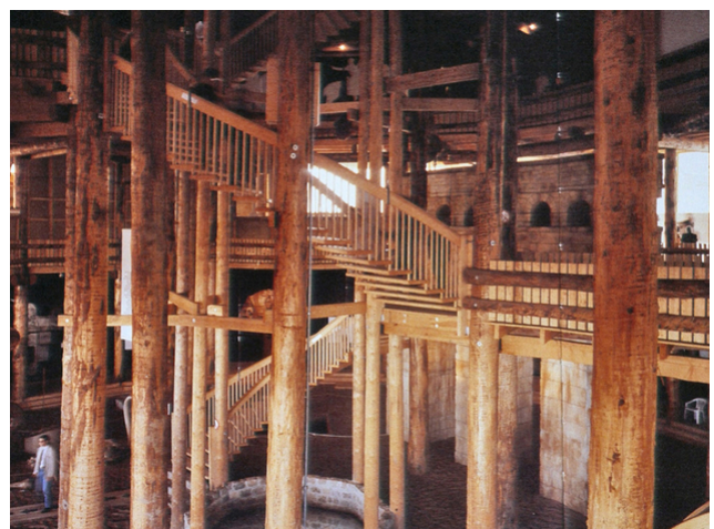
The interior of the tower
