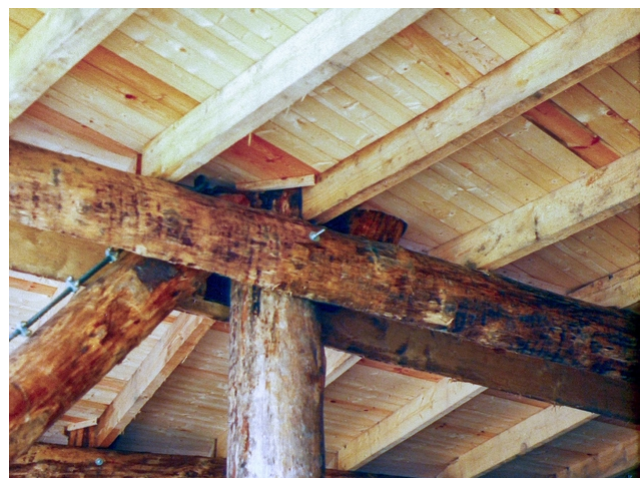
... and the application on the construction
