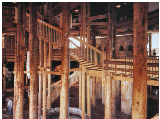
The interior of the tower
