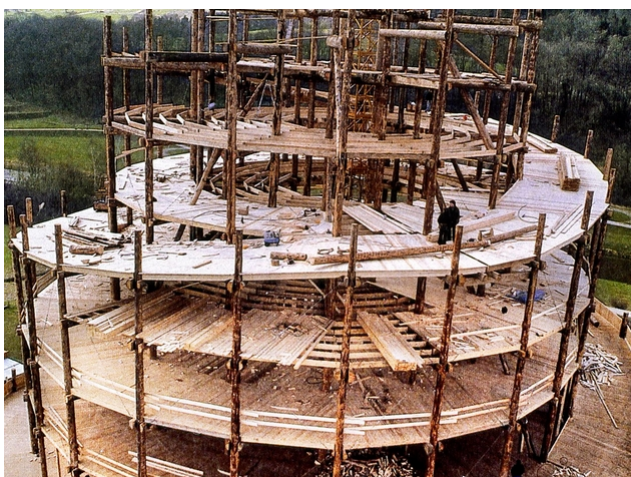
Tower in shell
