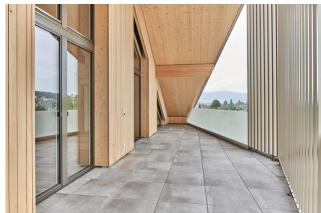
In the village center of Gretzenbach in the canton of Solothurn, a timber building with twelve apartments and a village store was built. The balconies cantilever over 3.5 meters - without any disruptive supports. An ingenious, suspended construction makes this possible.
