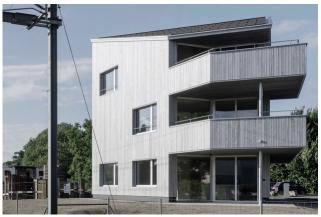
On Bachstrasse in Buchs in the canton of Aargau, a multi-family house was built in timber construction, which was originally planned as a reinforced concrete structure. The TS3 technology made it possible to change the material in the planning phase.
