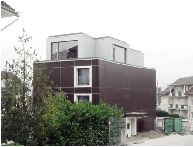
Exterior view street side from above
