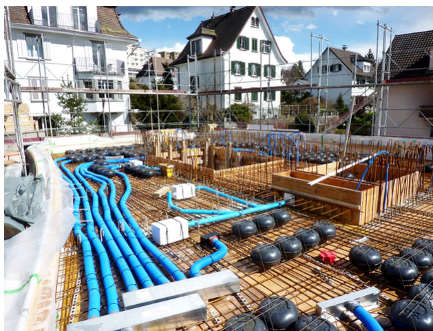
Concrete ceiling over ground floor shortly before concreting
