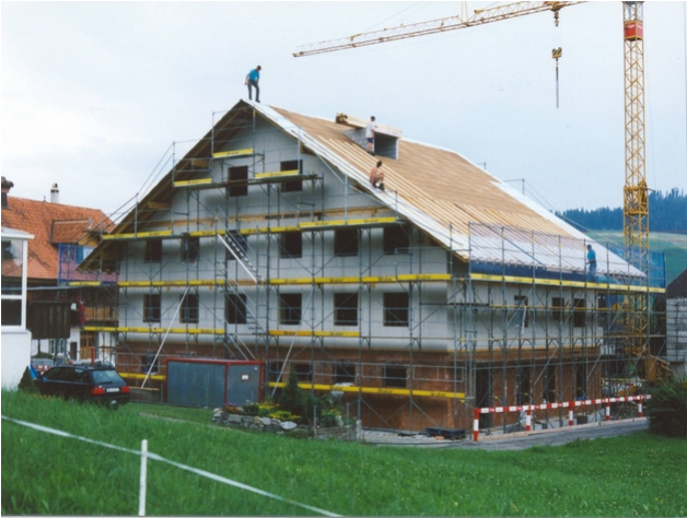
In the construction phase
