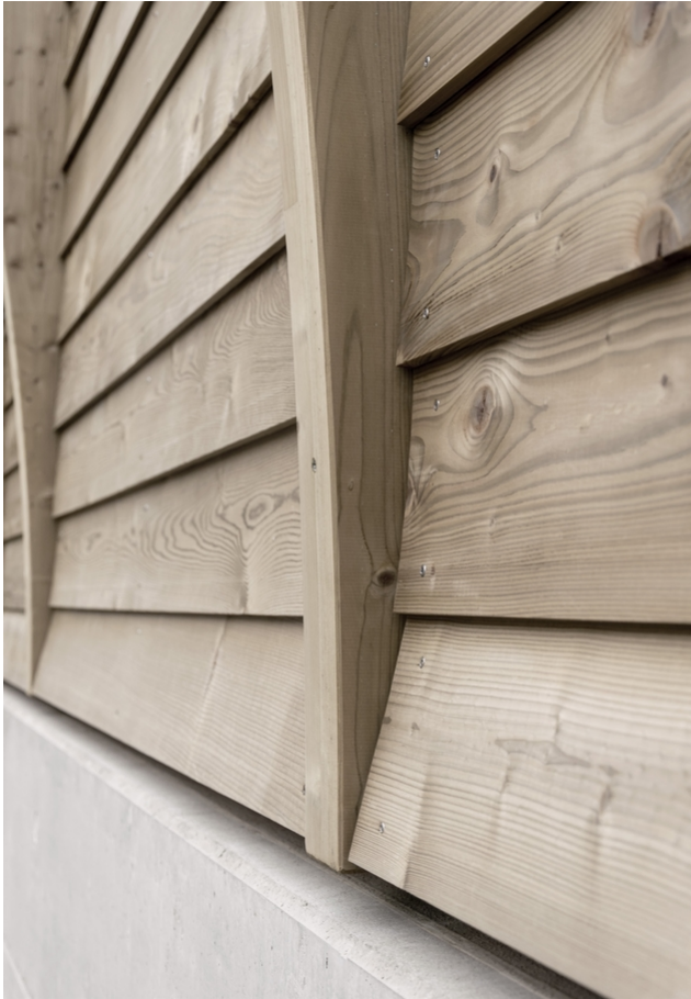
Detail of facade formwork
