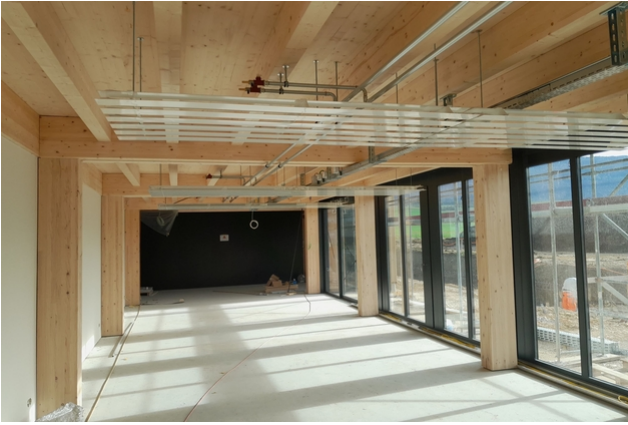
Interior view of the office area
