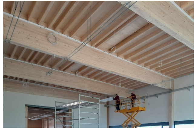
Construction of the hall ceiling
