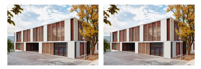
Wood characterizes the children's everyday school life at the Schachenmatten school building in Bonstetten. Built in 2015, the school building is a hybrid construction with concrete ceilings and load-bearing exterior walls made of wood. The example shows: Wood construction is also becoming increasingly important for public buildings.
