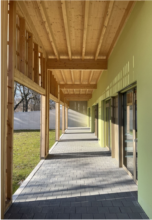
The portico with the visible joists
