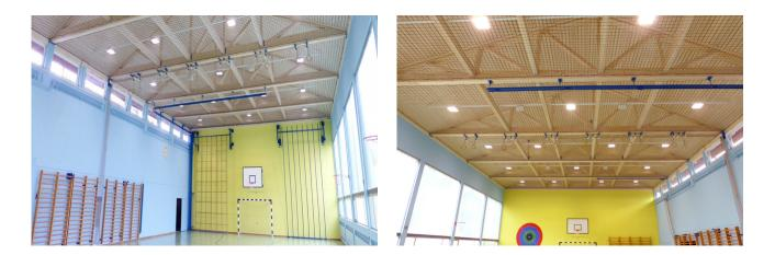
On behalf of the municipality of Bösingen, Timbatec AG carried out an expertise on the roof of the gymnasium. It showed that the structural safety of the supporting structure was no longer guaranteed.
