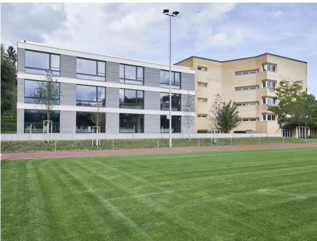
The newly designed surroundings of the school facility in Oberengstringen
