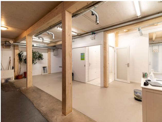
Central post-and-beam structure
