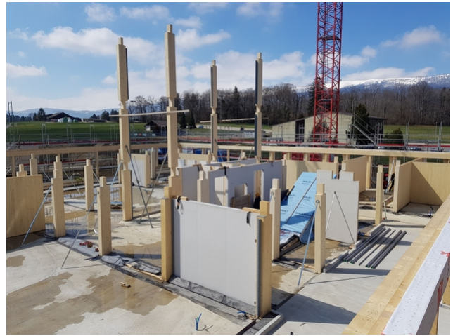
First floor under construction.
