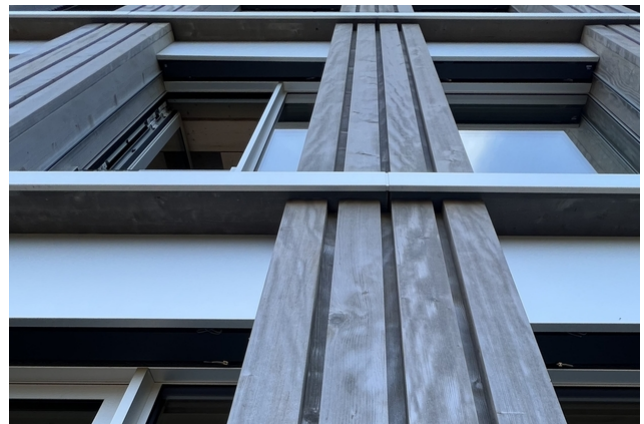
Wooden facade with surface treatment / Photos: luca da campo und École des Joncs in 2515 Prêles, Architektur: riforma architecture sa
