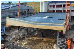
The new parking and cleaning area at the end of the day on Place de Chamblon was built with a wooden roof based on the origami principle. CLT and TS3 panels made this principle possible.
