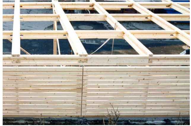
Finished car shelter
