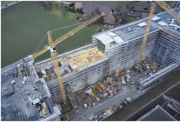
Aerial view during erection
