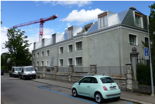
Exterior view in finished state
