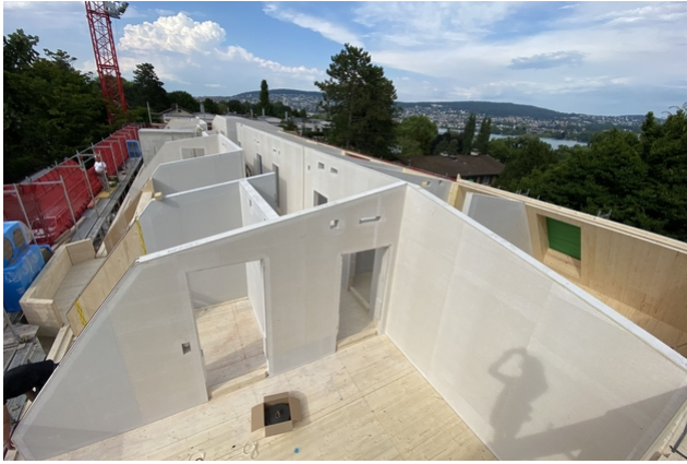
View directly into the element construction elevation
