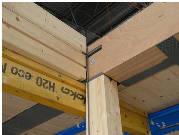
Beams made of beech wood
