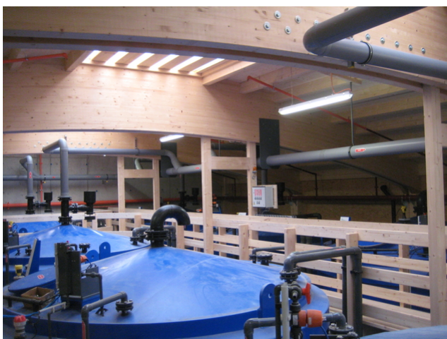
Hall de stockage zone 1
