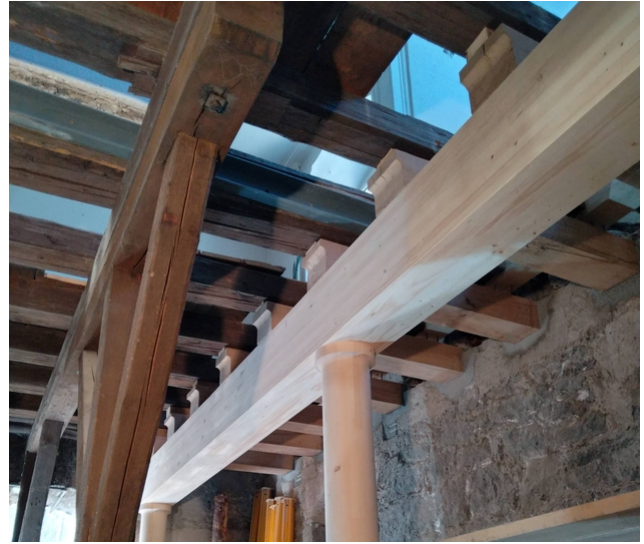
Renovation measures in the wine cellar
